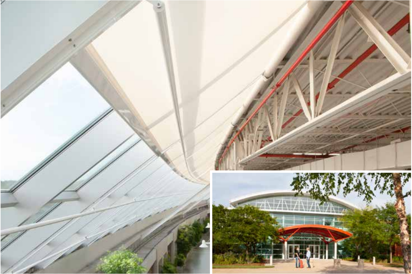
ABOVE: Custom Motorized Coupled FlexShade Systems with custom wheeled hem bars in side tracks and intermediate rollers, Fabric is Mermet E-Screen 5% White Linen. INSET: Oustide Herman Miller Inc. manufacturing, Holland, MI Dealer: Triangle Window Fashions., Photography: Barry Rustin
